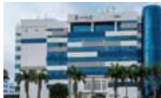
10 Changi South Lane
